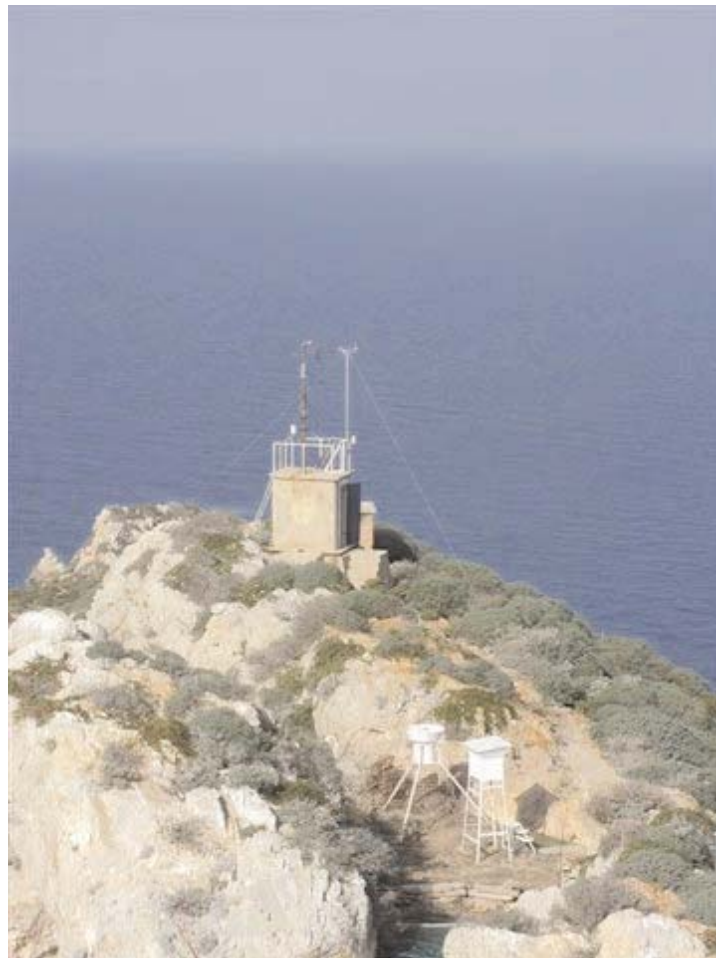
Meteorological station Palagruža, MHS, Croatia
